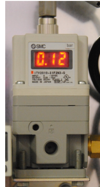
Automatic air pressure regulator
